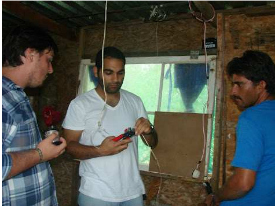
Omid and Graeme helping to install a solar panel.
