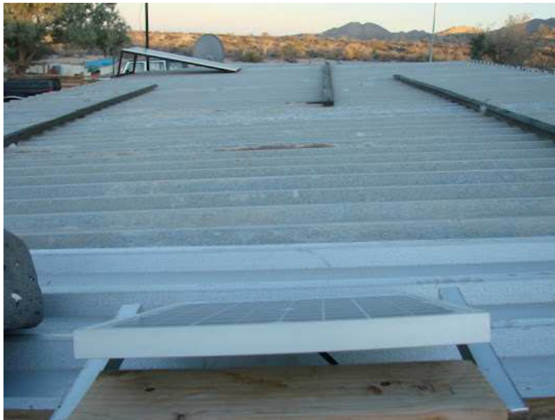
One of the new solar panels installed on the roof with a home-made base which will allow the family to move the panel to follow the sun at different times during the day.
